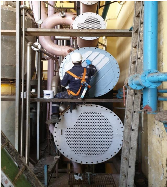
Application of high-temperature epoxy coating, Belzona 1391T to protect tube sheet Engineering a More Environmentally Sustainable Future
